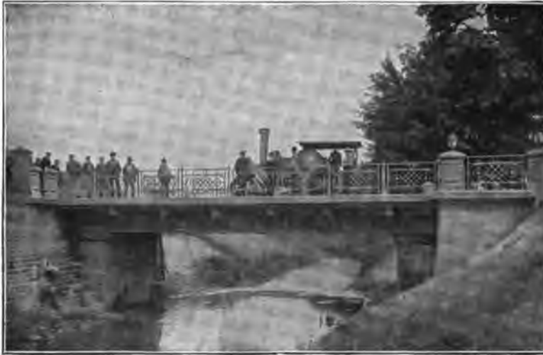
FIG. 275.—Hornback Bridge near Zweibrücken.
