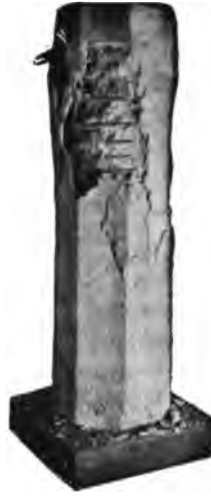
FIG. 73.—Spalling of the outer concrete shell.
