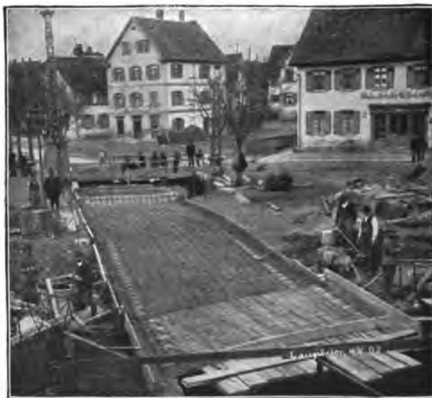
FIG. 271.—Laufbach Bridge in Laupheim. Placing Reinforcement.
