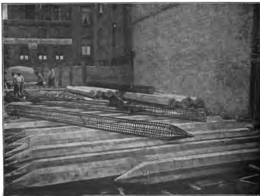
FIG. 267.—Behrend Building, Kiel. Stock of finished piles and some reinforcement units.
