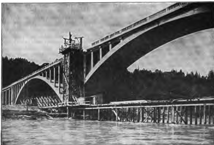
FIG. 301.—View under the arch over the right-hand stream.
