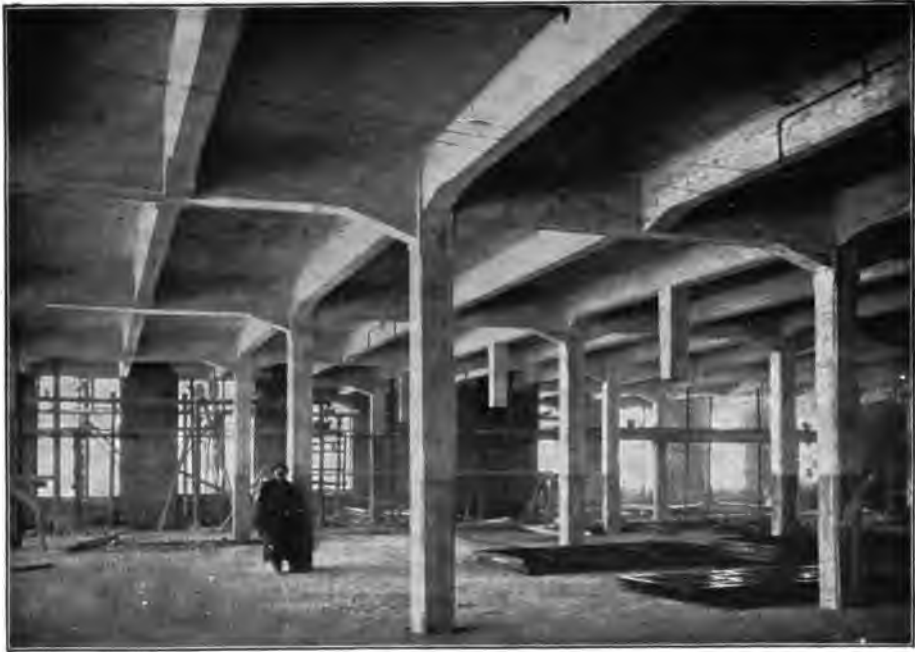
FIG. 208.—Hanging columns for the carrying of shafting in the Speyer cotton mill on the Rhine.
