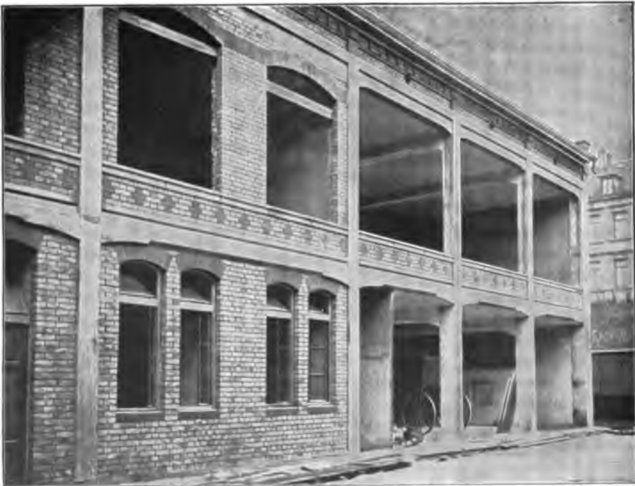
FIG. 209.—Office building of Wayss & Freytag, Neustadt-on-the-Hardt.
