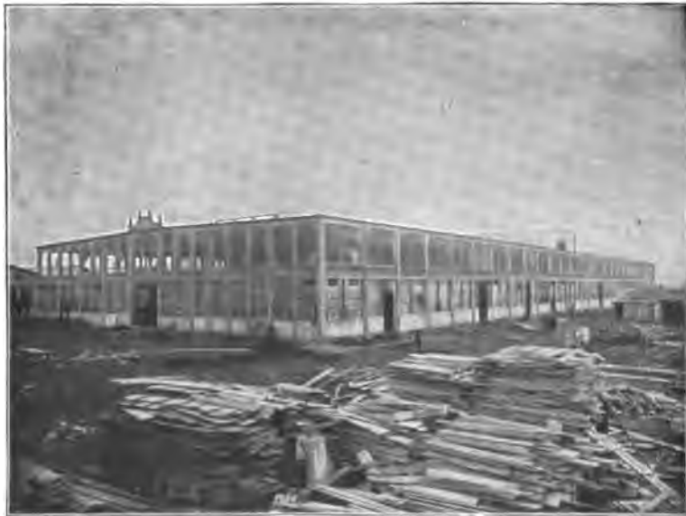
FIG. 213.—Factory of the Daimler Motor Co. in Unterturkheim near Stuttgart.
