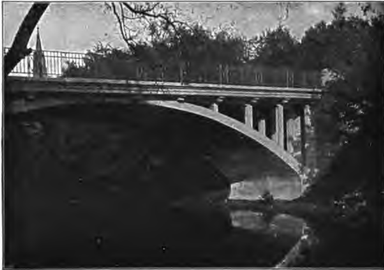
FIG. 305.—Nagold Bridge near Caln (Württemberg).
