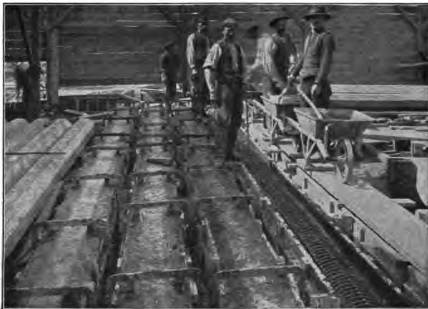
FIG. 266.—Factory in Metz. Placing concrete in pile forms.
