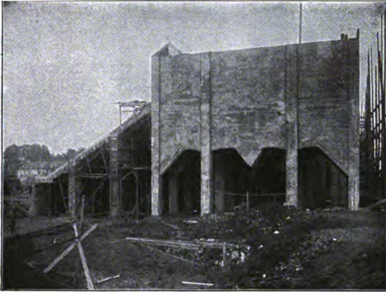
FIG. 332.—Maizière ore pockets. 178 m. (583 ft.) long.
