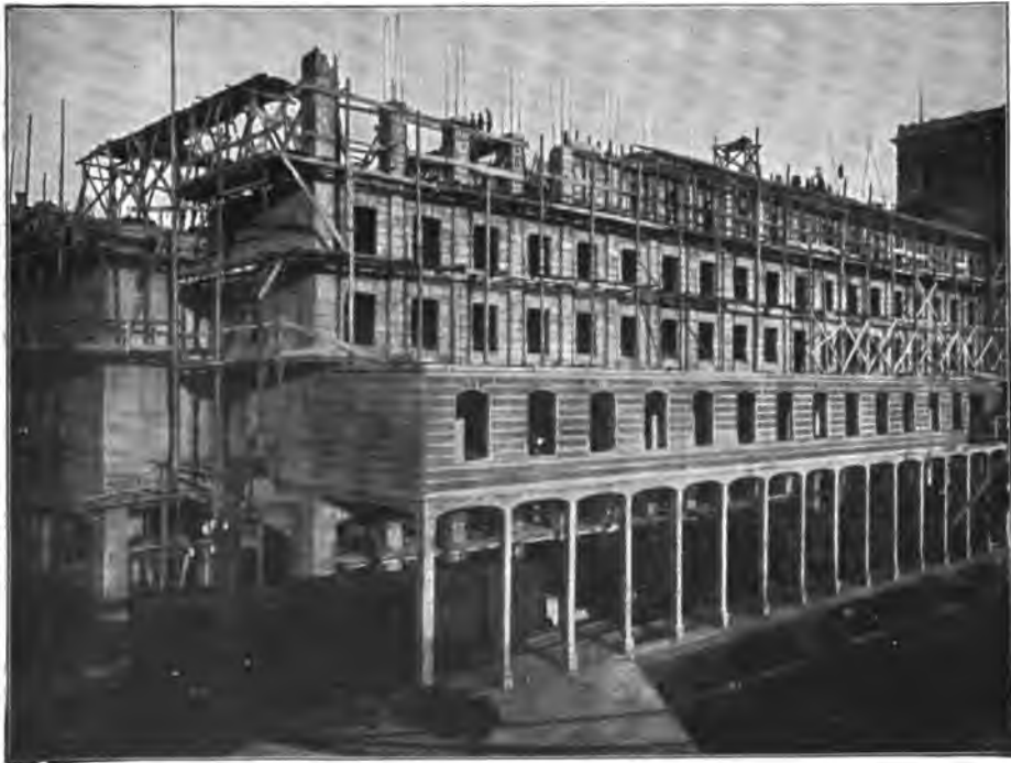
FIG. 341.—View of the silo in Genoa with the colonnade toward the harbor.
