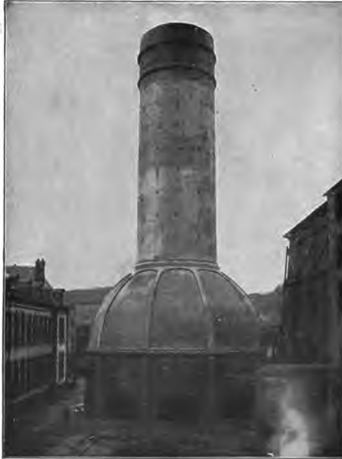
FIG. 346.—Cooling tower of the Differdingen Steel Works.
