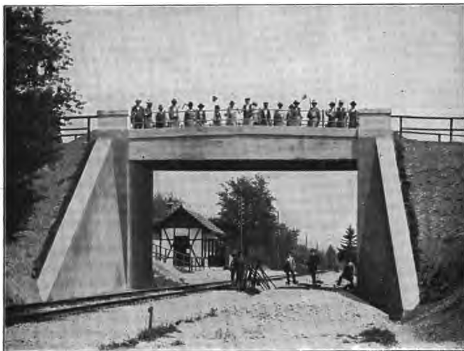
FIG. 282.—Highway Bridge in Grimmelfingen near Ulm. Tested to 450 \text{ kg/m}^2 ( 92 \text{ lbs/ft}^2 ) with gravel; deflection 0.2 mm. (0.008 in.).
