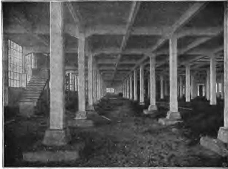
FIG. 212.—Foundations, Daimler motor factory near Stuttgart.
