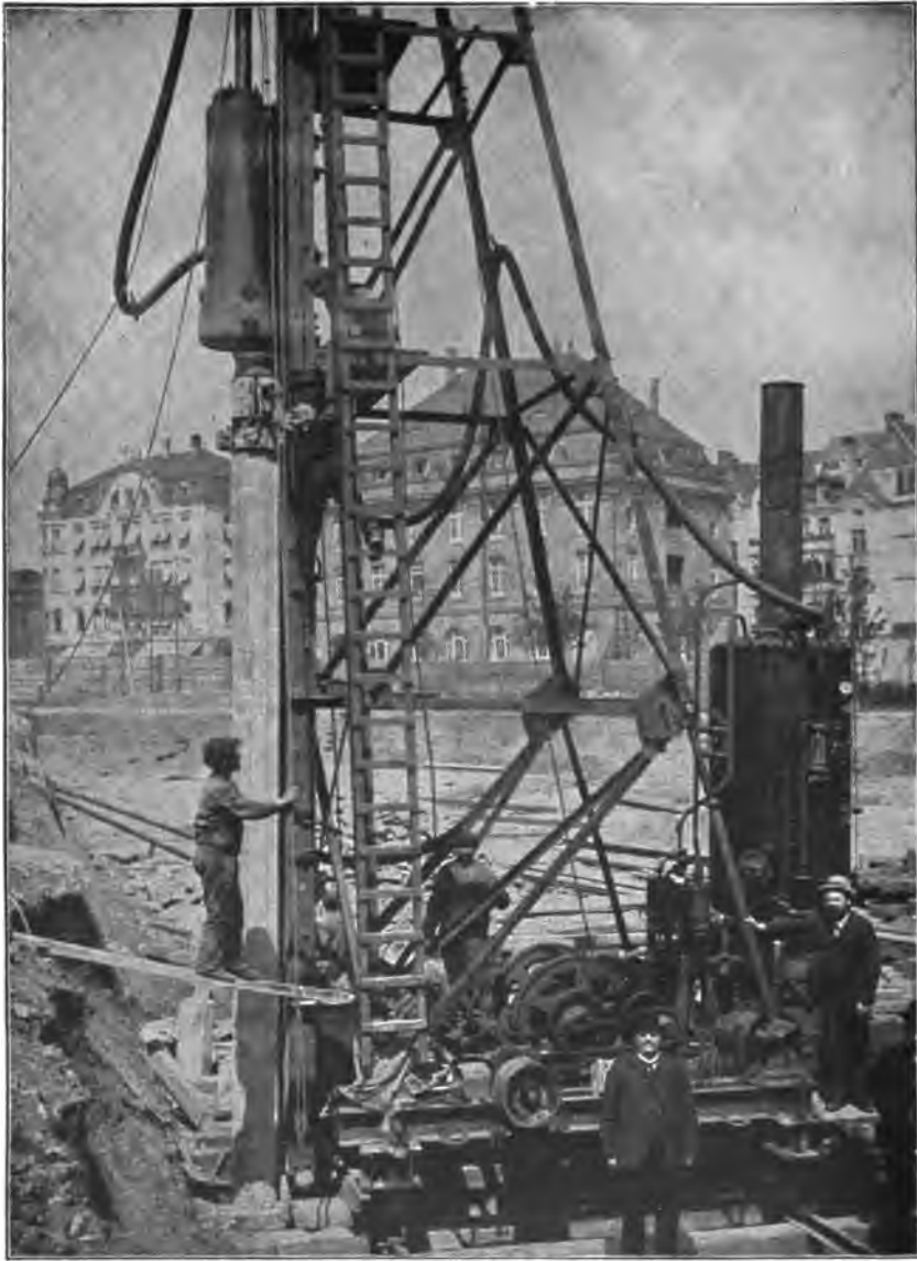
FIG. 269.—Business building in Metz. Driving piles.
