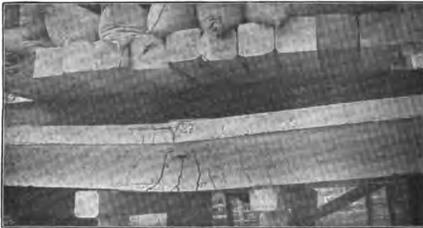
FIG. 160.—Beam X, under the breaking load.
