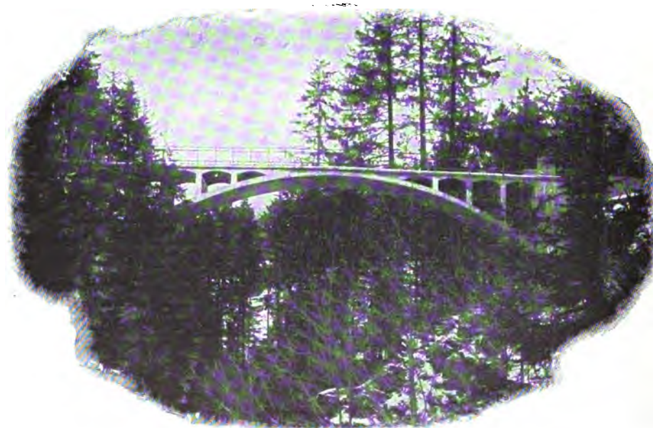
FIG. 292.—Highway bridge in Gunzesried (Allgäu). Span 32 m. (105 ft.).
