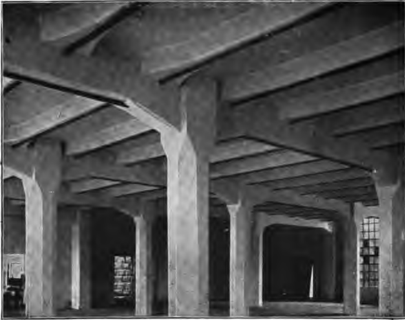
FIG. 229.—View of a floor in the Singer Manufacturing Co. factory showing widening of the beams where they intersect the girders. Columns of béton fretté.
