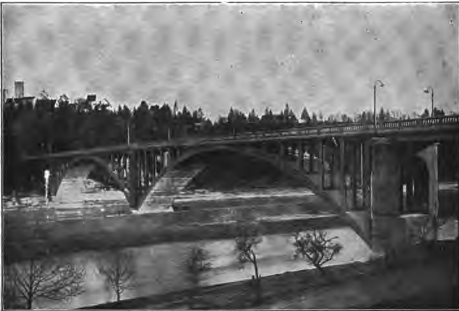
FIG. 295.—Highway bridge over the Isar near Grünwald.
