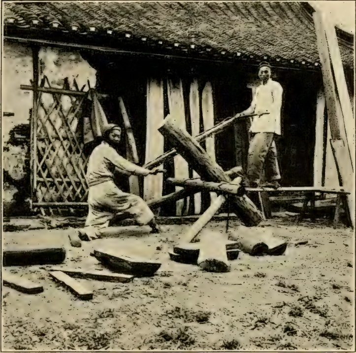
FIG. 28. - Usual method of sawing lumber in China.
